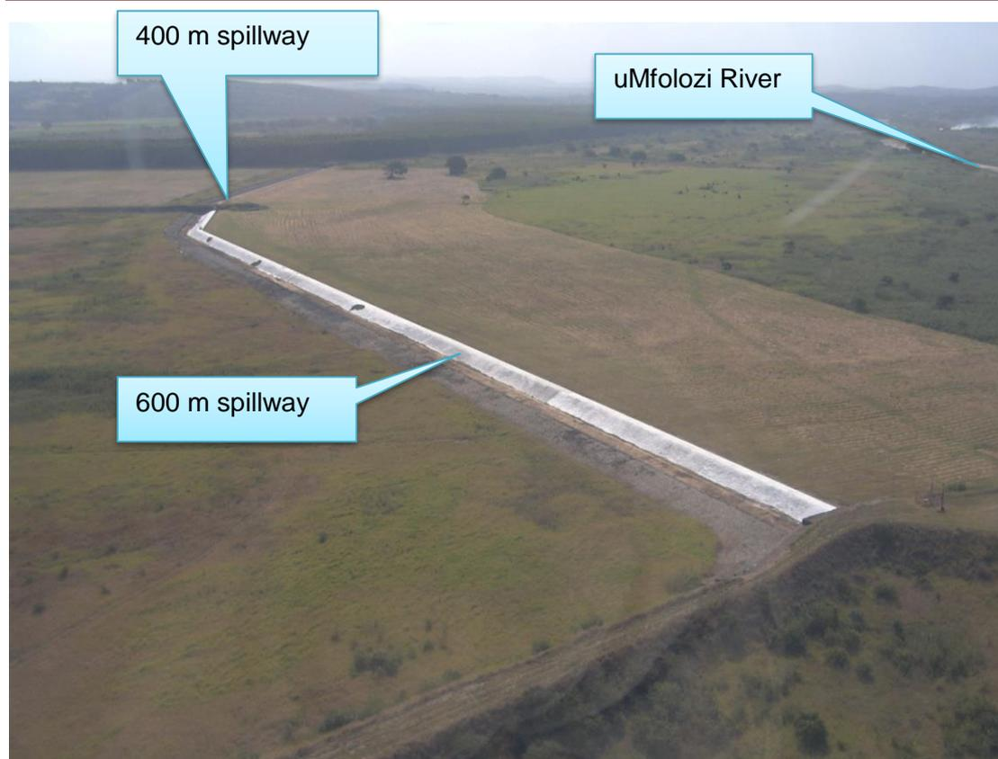
**Figure 4.2.1-1** Aerial view of the 600 m and 400 m spillways of the uMfolozi River Diversion viewed from the south
